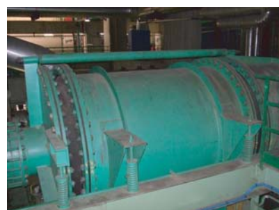
TPA with DILATOFLEX® DN 2500
